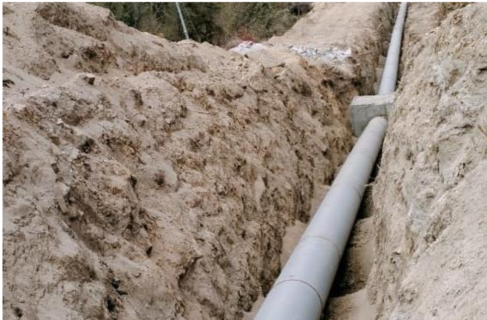
Figure 7-24: Penstock Pipe Anchor Block VAB 03
