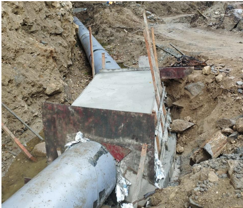
Figure 7-18: Headrace Anchor Block HAB 05
