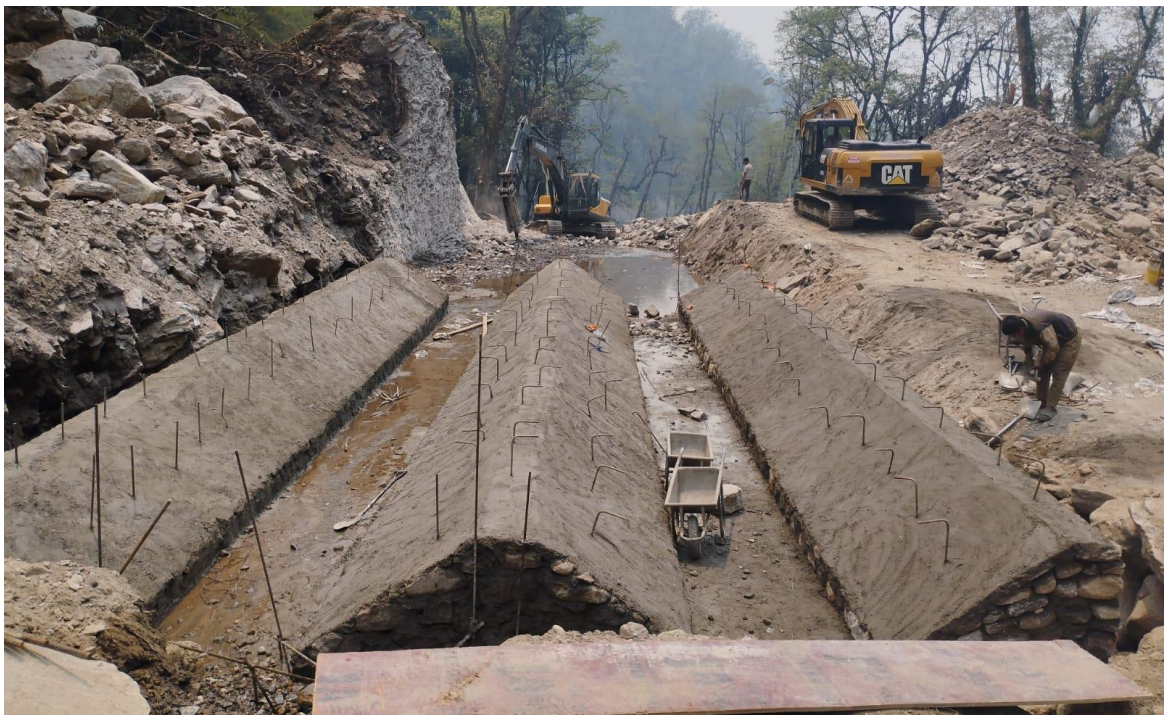
Figure 7-13: Stone Masonry at Desander
