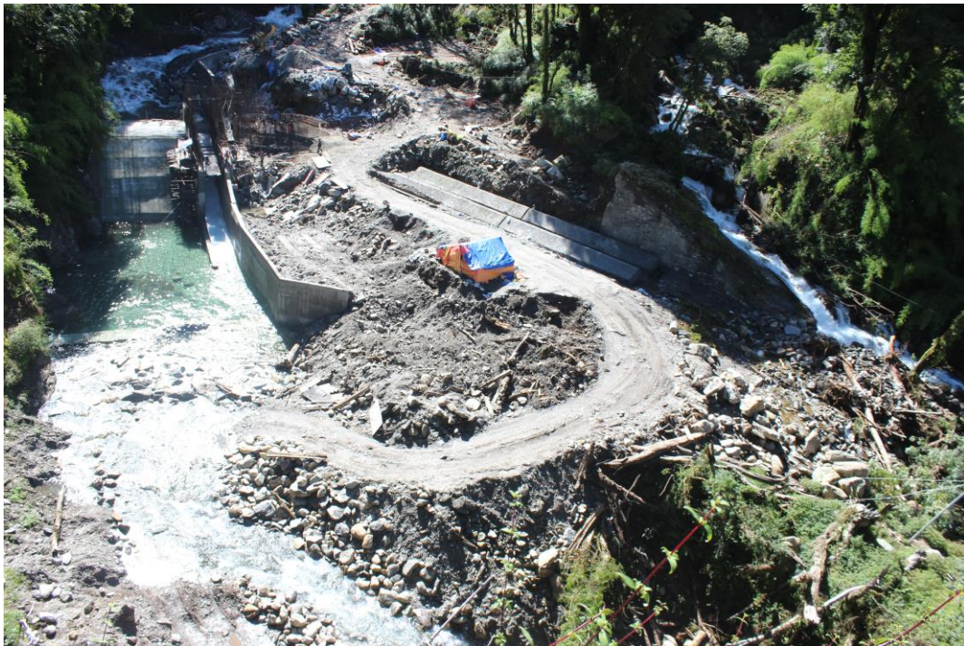
Figure 7-11: Work Progress at Weir, Stilling basin and Undersluice including floodwall and protection works
