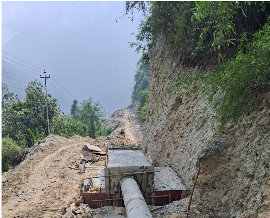
Figure 7-26: Penstock Pipe Anchor Block CAB20
