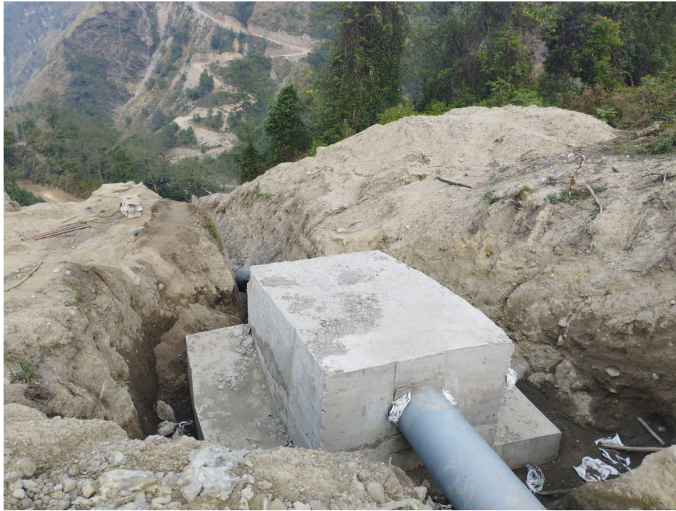
Figure 7-32: Penstock Pipe Anchor Block VAB10
