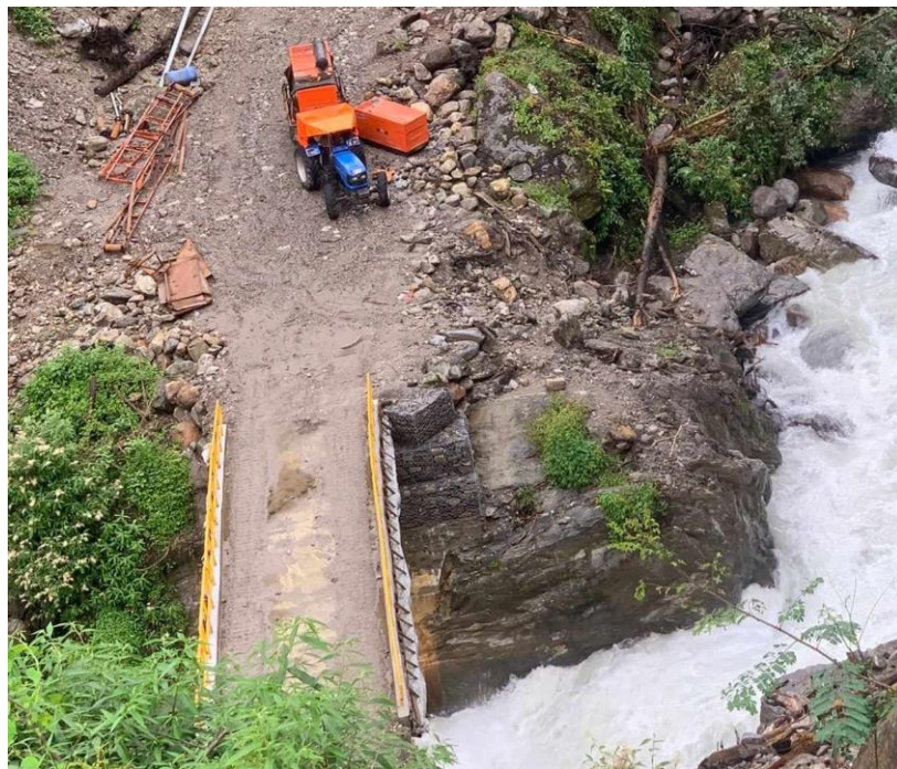
Figure 7-3 Composite steel girder with RCC deck bridge work on progress
