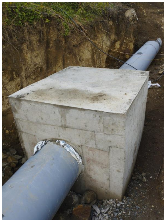
Figure 7-25: Penstock Pipe Anchor Block VAB 04
