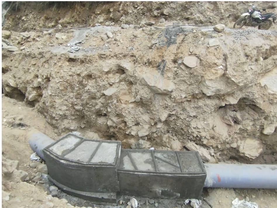
Figure 7-16: Headrace Anchor Block HAB 03 and Road crossing
