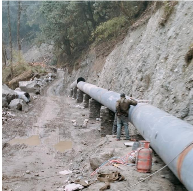
Figure 7-14: Headrace Pipe erection near HAB 02
