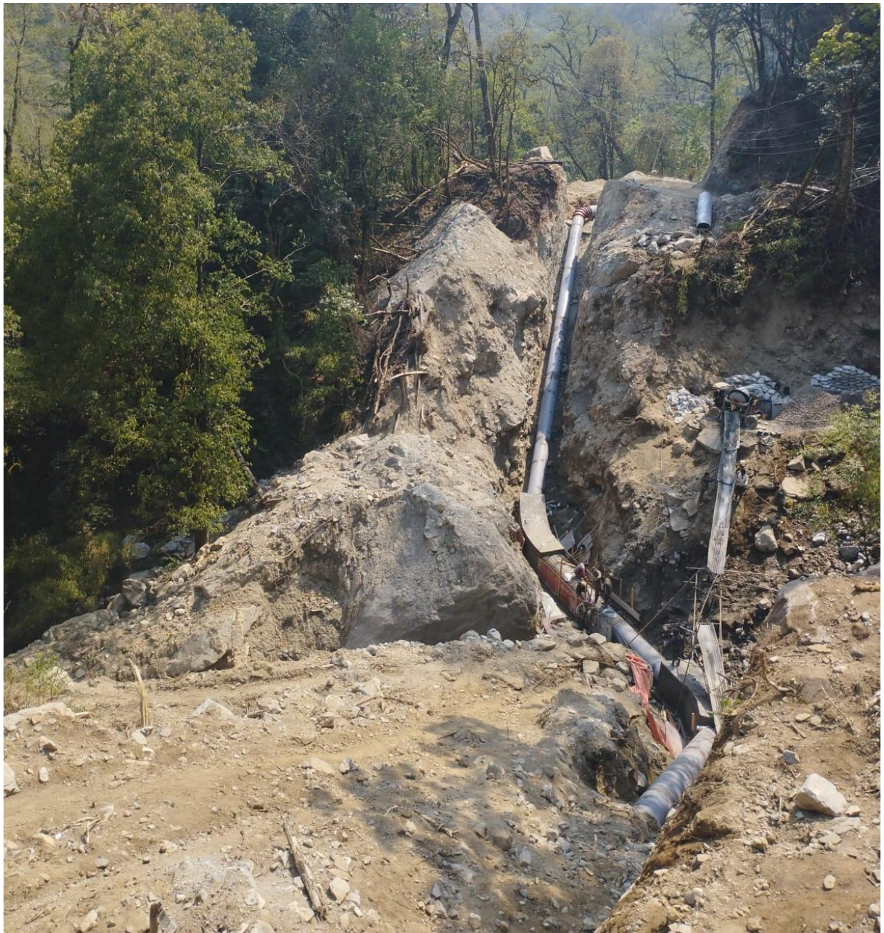
Figure 7-15: Headrace Anchor Block CAB3, CAB4, CAB5 and CAB6 including Siphon crossing
