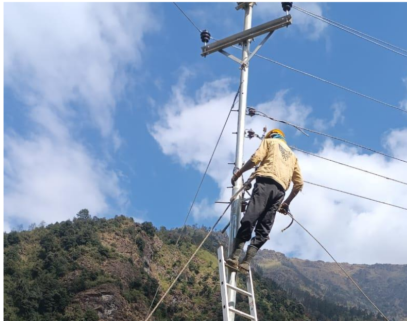
Figure 7-8: Electric Pole and accessories erection for construction power
