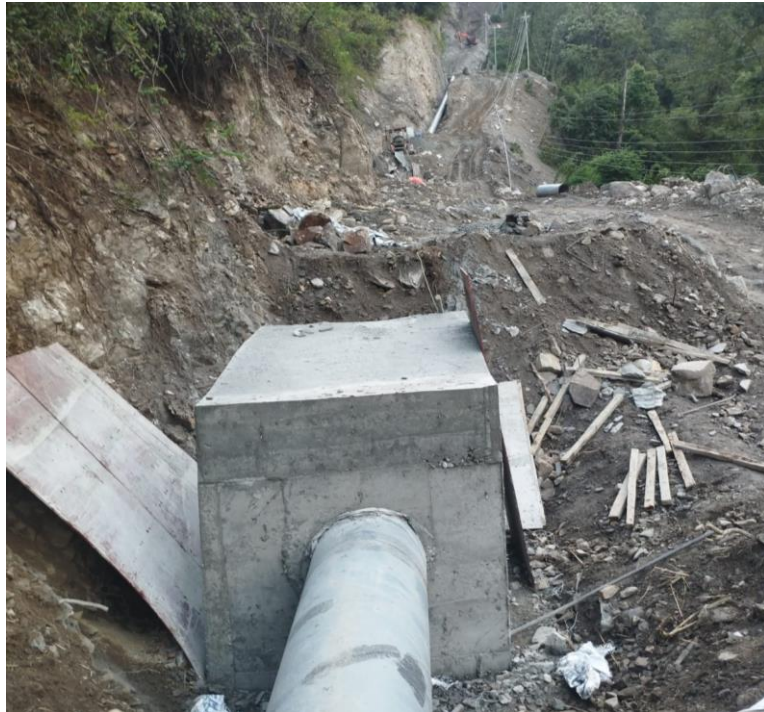
Figure 7-28: Penstock Pipe Anchor Block VAB 06
