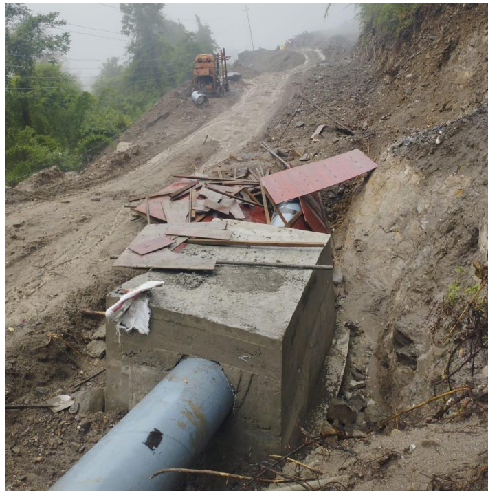
Figure 7-27: Penstock Pipe Anchor Block CAB 21
