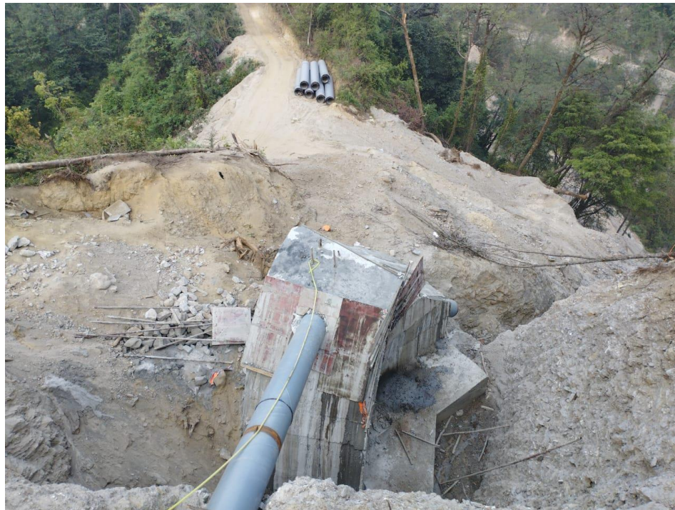
Figure 7-33: Penstock Pipe Anchor Block CAB23
