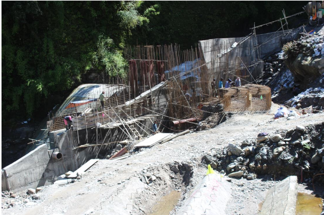
Figure 7-12: Work progress in Intake, Gravel Trap, Flushing Pipe and Gate, Approach canal
