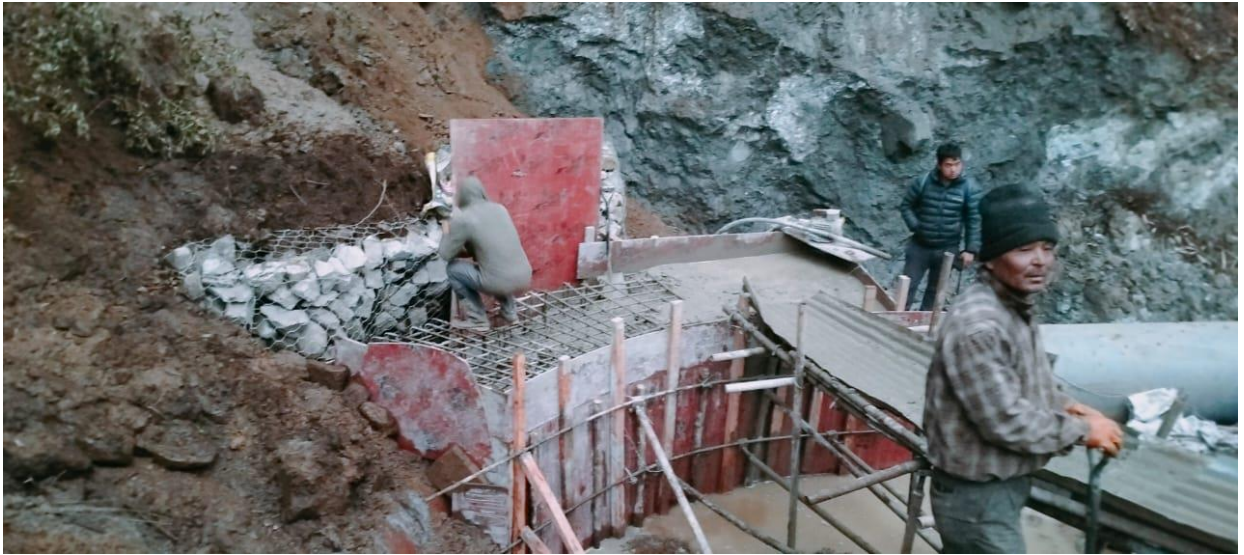
Figure 7-21: Headrace Anchor Block HAB08
