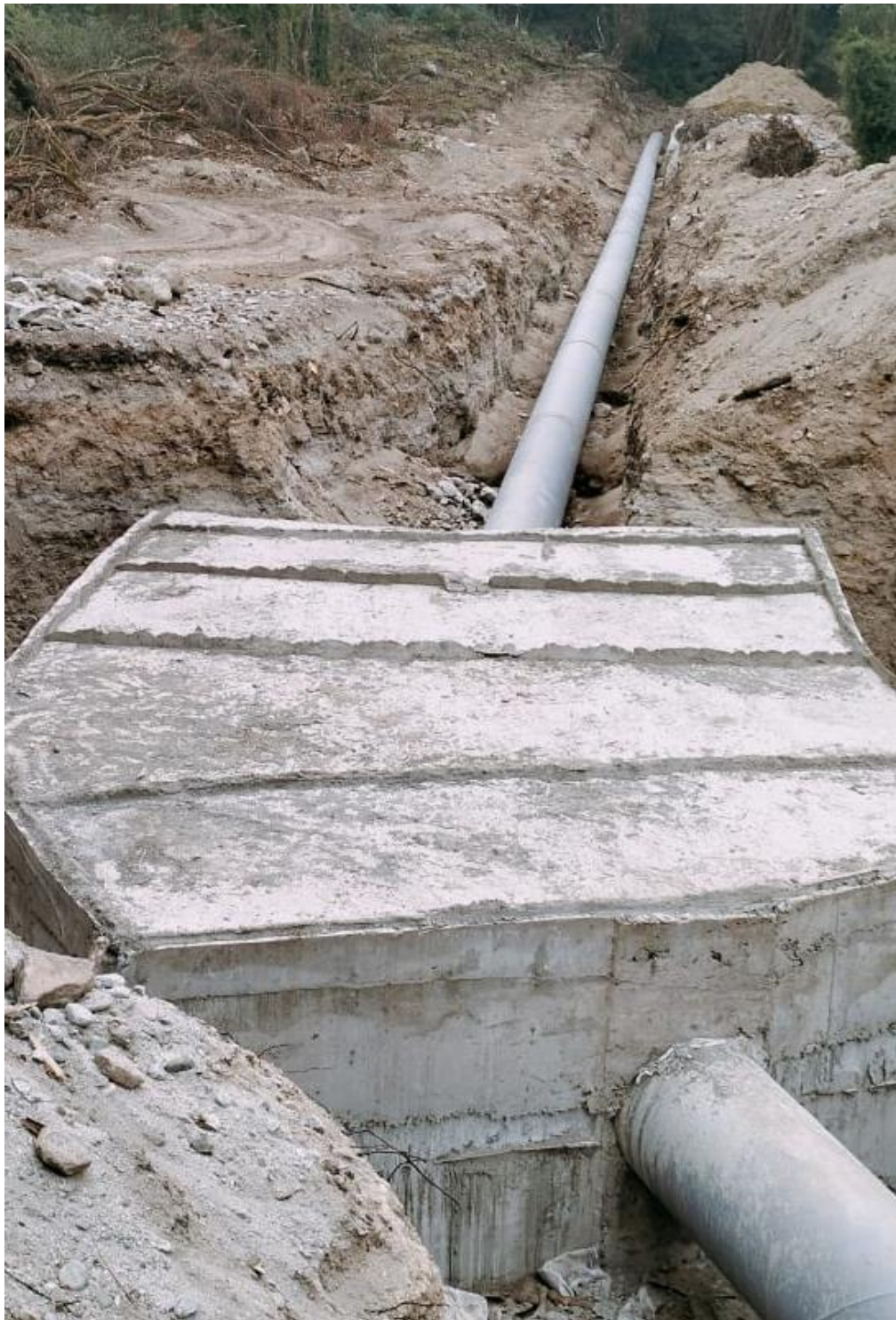
Figure 7-23:Penstock Pipe Anchor Block CAB 14
