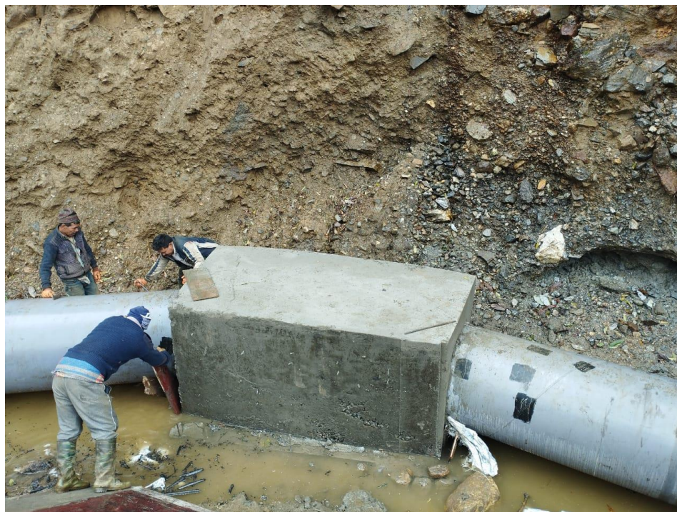
Figure 7-17: Headrace Anchor Block HAB 04
