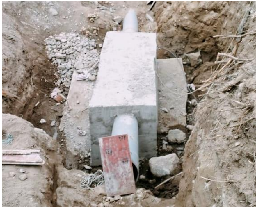
Figure 7-31: Penstock Pipe Anchor Block VAB 09
