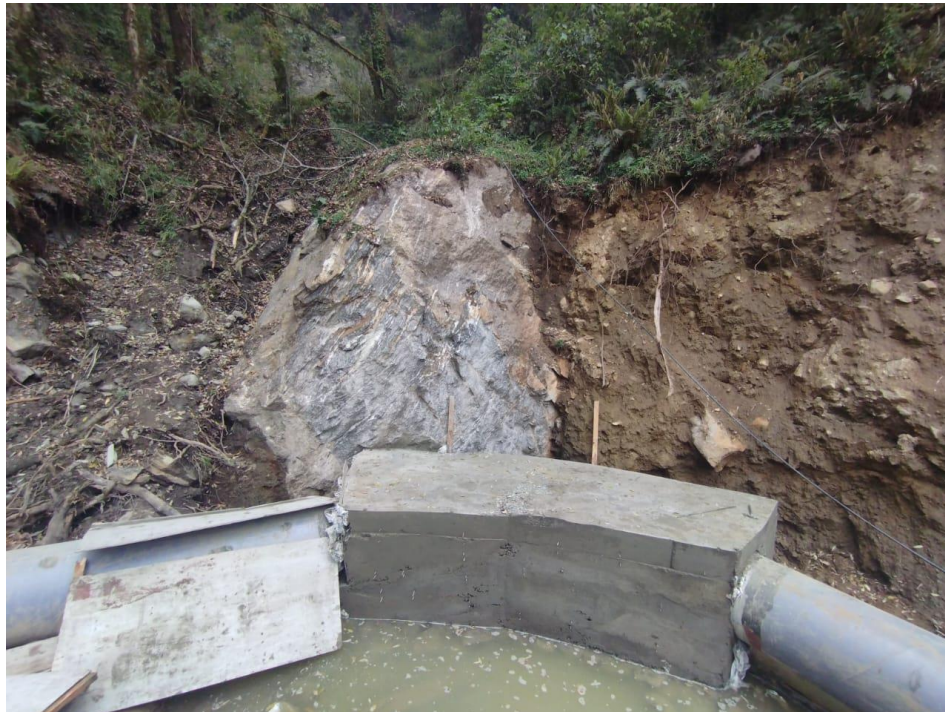
Figure 7-19: Headrace Anchor Block HAB 06
