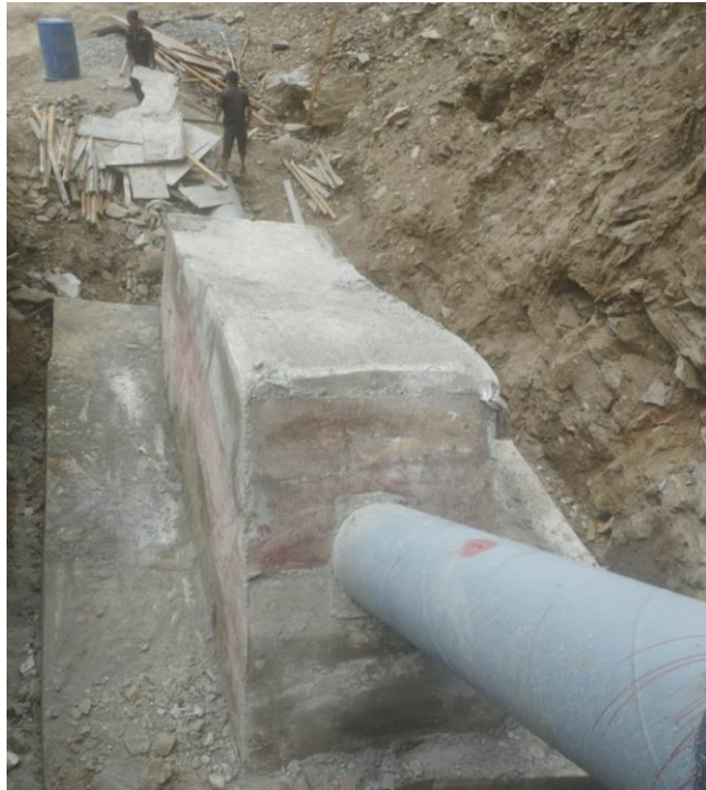
Figure 7-30: Penstock Pipe Anchor Block VAB 07
