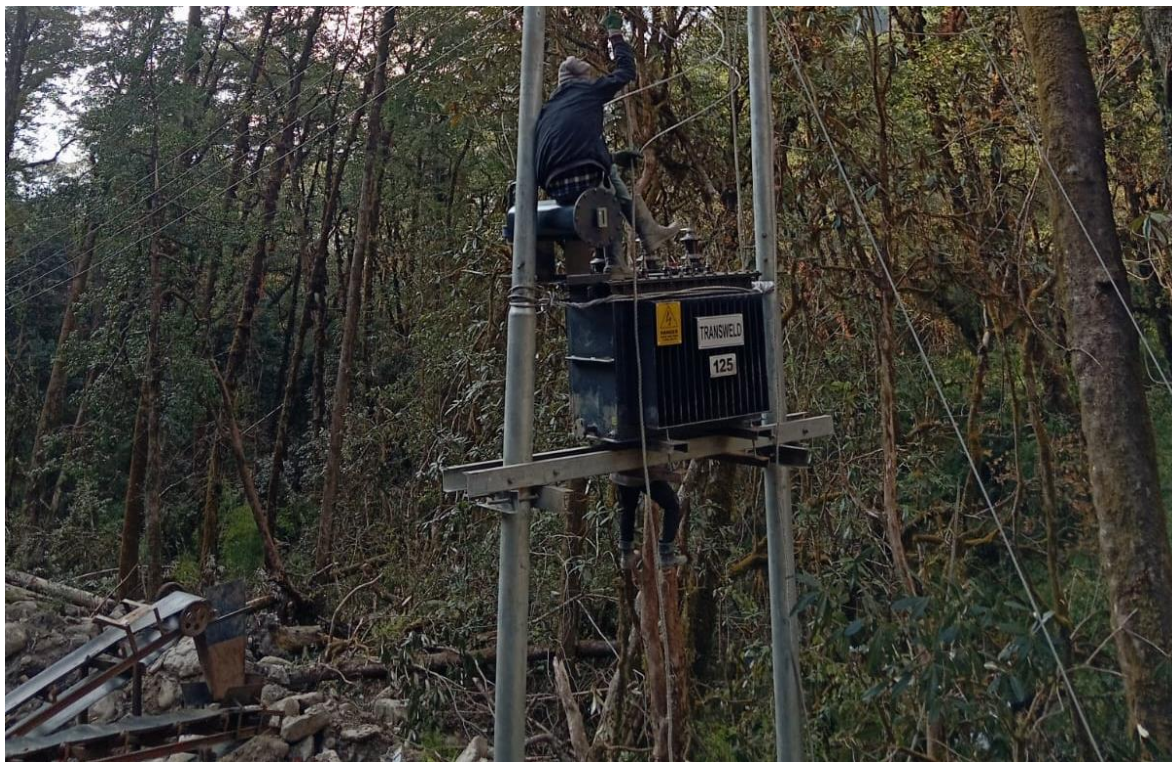
Figure 7-9: Transformer Installation at Intake
