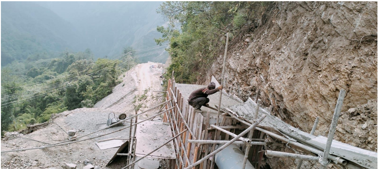
Figure 7-29: Penstock Pipe Anchor Block CAB 22
